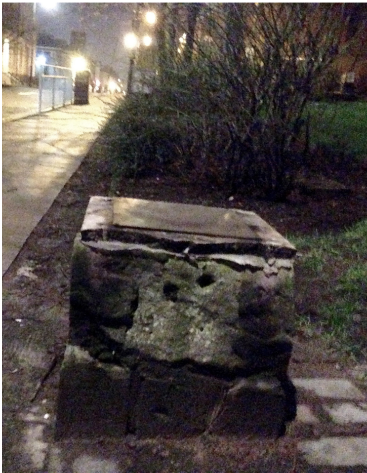
Here I have noted the obvious absence of one of the Mackintosh style beacons, the hole has simple been covered up with plate metal. This points to a lack of systematic maintenance, and perhaps flaws in the light fittings themselves.
