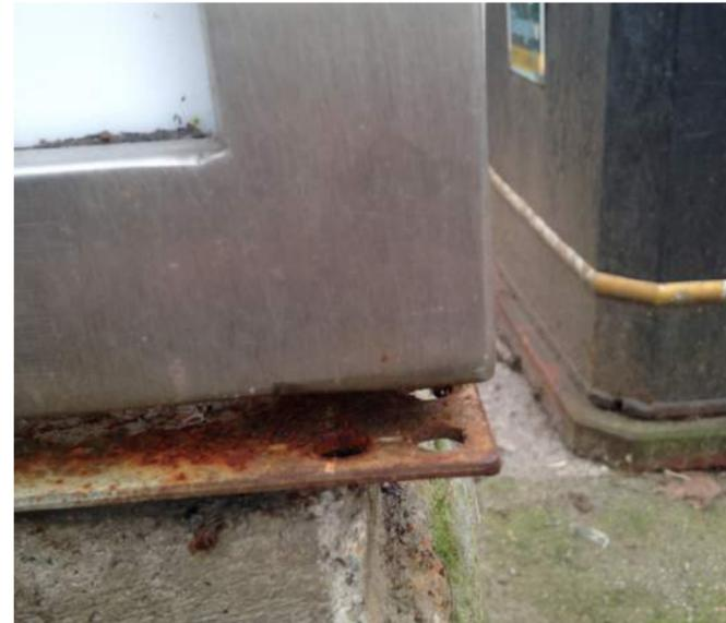
Most of the unsteadiness of the box is caused by missing bolts in the bottom sheet. Often this is because the metal has rusted though, but can be put down to lack of maintenance in other cases. Frames 100% locked down are impressively steady.
