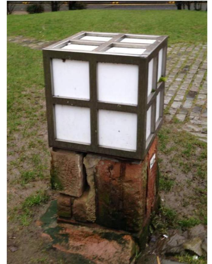
The current light was implemented in the redevelopment 25 years ago. Technical specifications are at the moment not apparent, and as a class, we haven't seen it being turned on. From what I can identify through observation, the box is constructed from sheet metal, with white plastic inserts.
